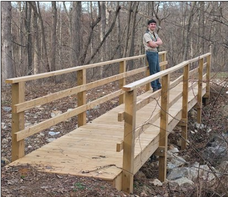
Jacob Cornwell stands on the bridge constructed for his Eagle Scout project.
