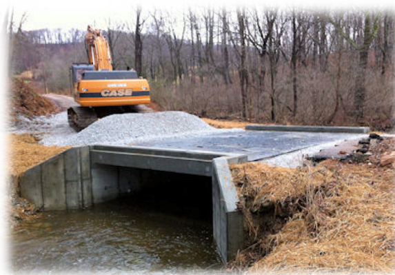
Newly installed box culvert on Sunny Slope Road.
