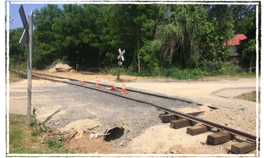
Mt. Airy Road: reconstruction of railroad crossing
